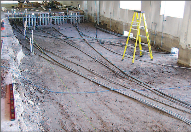
Compacted top-soil over a duct bank in preparation for electrical switchgear and a 12,000-gallon fuel tank to be housed inside an explosion-proof room.
